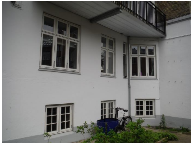
Renoveret underfacade mod gård
