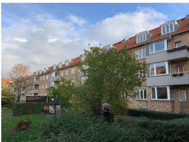
Facade mod gård.
